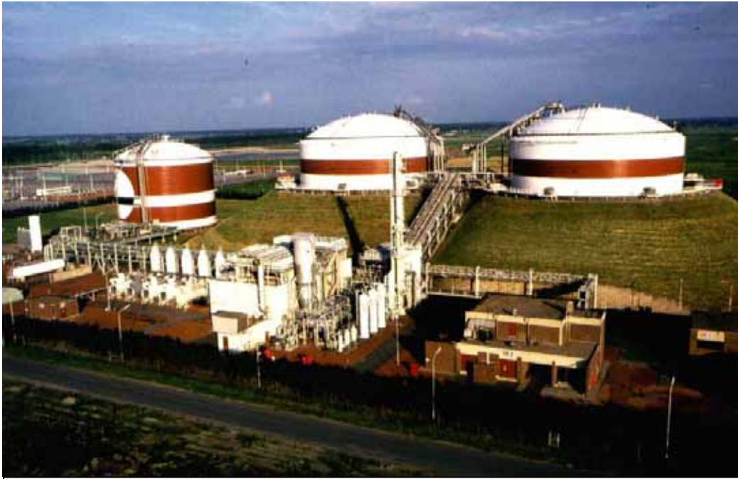
Figure (1) LNG Peak Shaving Plant in Belgium
